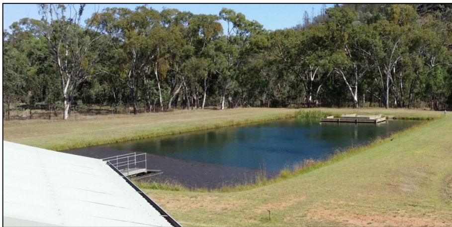
Figure 4-5: Sedimentation Lagoon 1 Nearing Capacity
