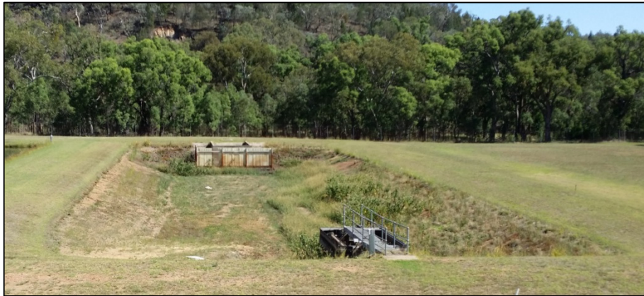
Figure 4-4: Sedimentation Lagoon 2 Offline for Drying
